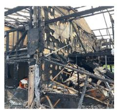
Photographs clearly showing combustible plywood cladding to the lower floor, plywood sheet & UPVC cladding spanning the party wall line to the upper floor, no insulation is present, also fire damage to remains of the plywood sheeting indicating surface fire spread via this route. Inspections into these areas were carried out.
