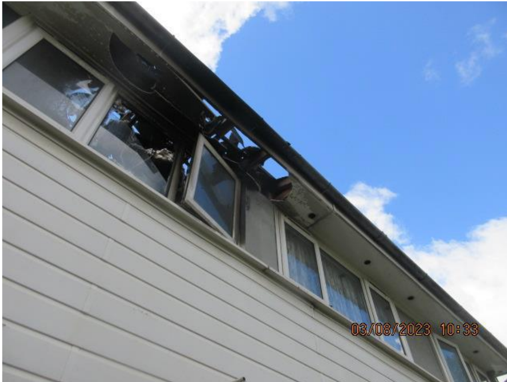
15. At the front showing the area spanning the party wall between 13 (on the left) and 15. The uPVC eaves soffit board of no 13 has been damaged but that of 15 is intact.
