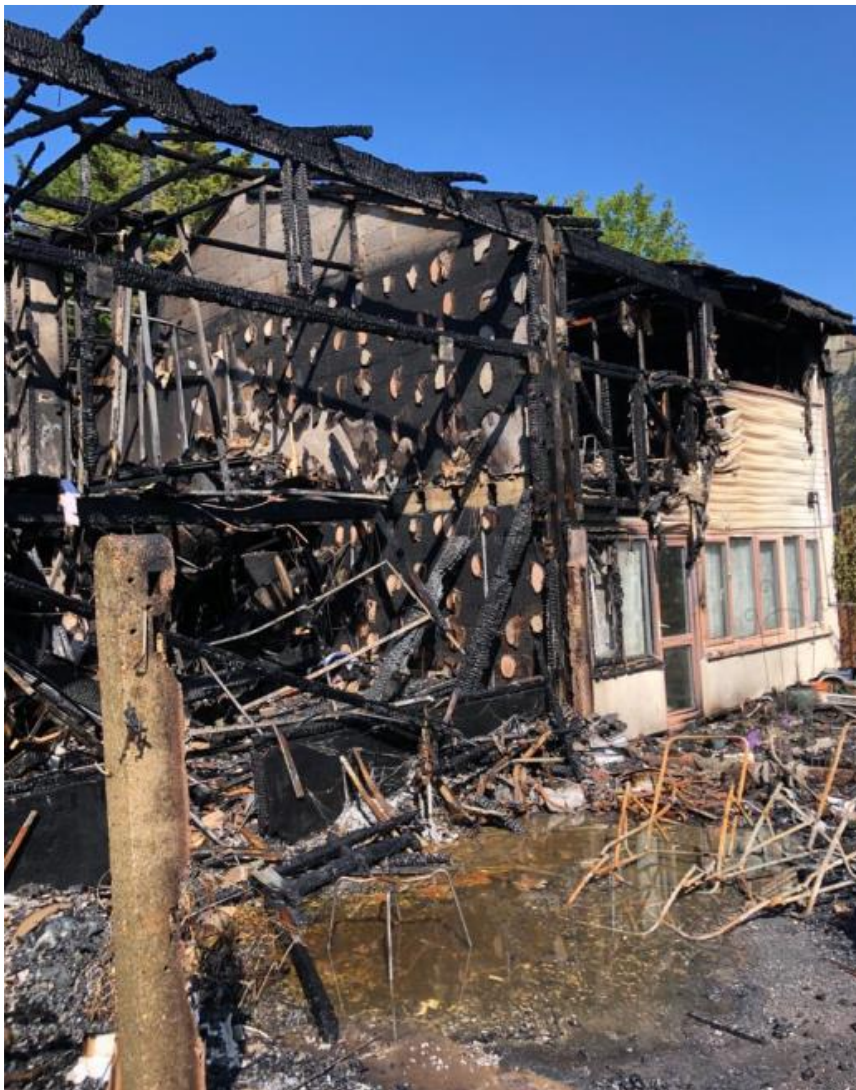
9. A view from the garden at the rear of no 9. The timber fence between the yard of 11 and the garden of 9 has been consumed by fire. The arrow indicates what appears to be a section of non-combustible board.
