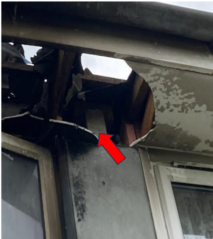
15. At the front showing the area spanning the party wall between 13 (on the left) and 15. The uPVC eaves soffit board of no 13 has been damaged but that of 15 is intact.
