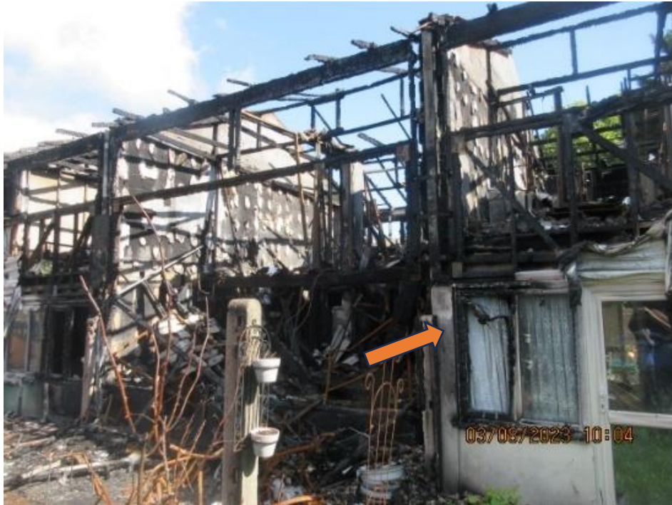
9. A view from the garden at the rear of no 9. The timber fence between the yard of 11 and the garden of 9 has been consumed by fire. The arrow indicates what appears to be a section of non-combustible board.
